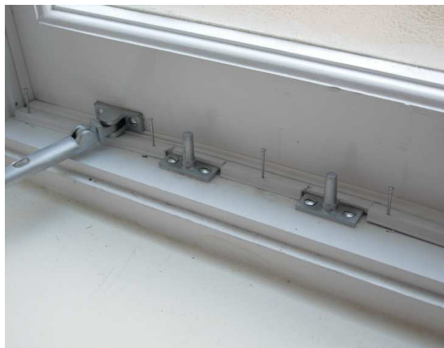
Examples of fitting Retro B strips to casement windows
