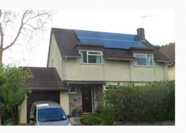
A 3 kw PV array which will provide on average 2,600 kWh a year requires 20 metres squared area with a cost of £4000. This house uses about the same quantity of electricity but note the mismatch of summer vs winter for generation vs consumption
