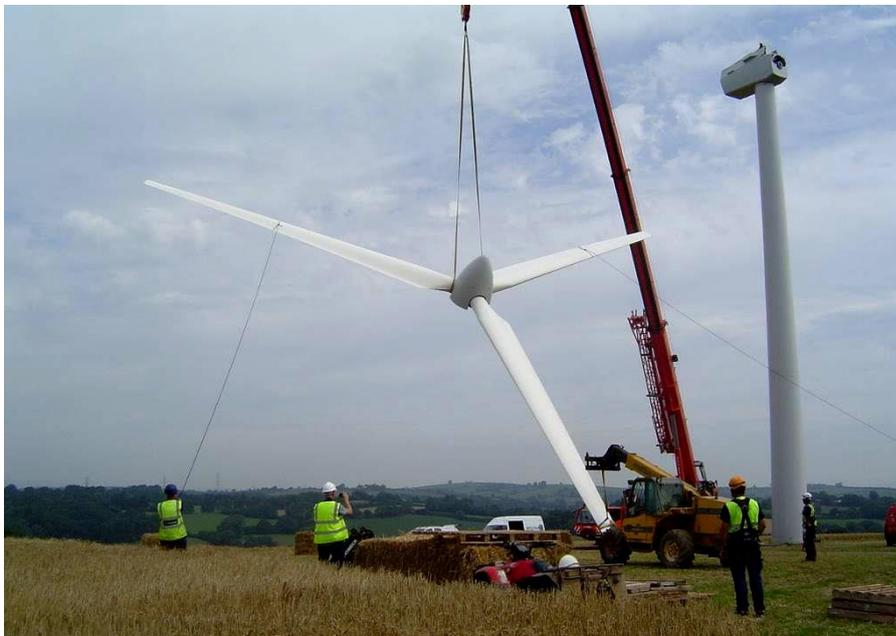
*The final stage of the V27 being assembled 23 August 2014*
